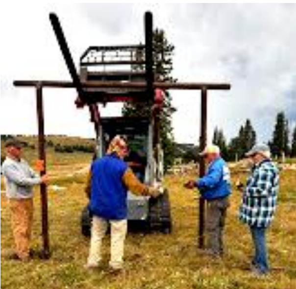
Measuring, leveling & perfect placement!
